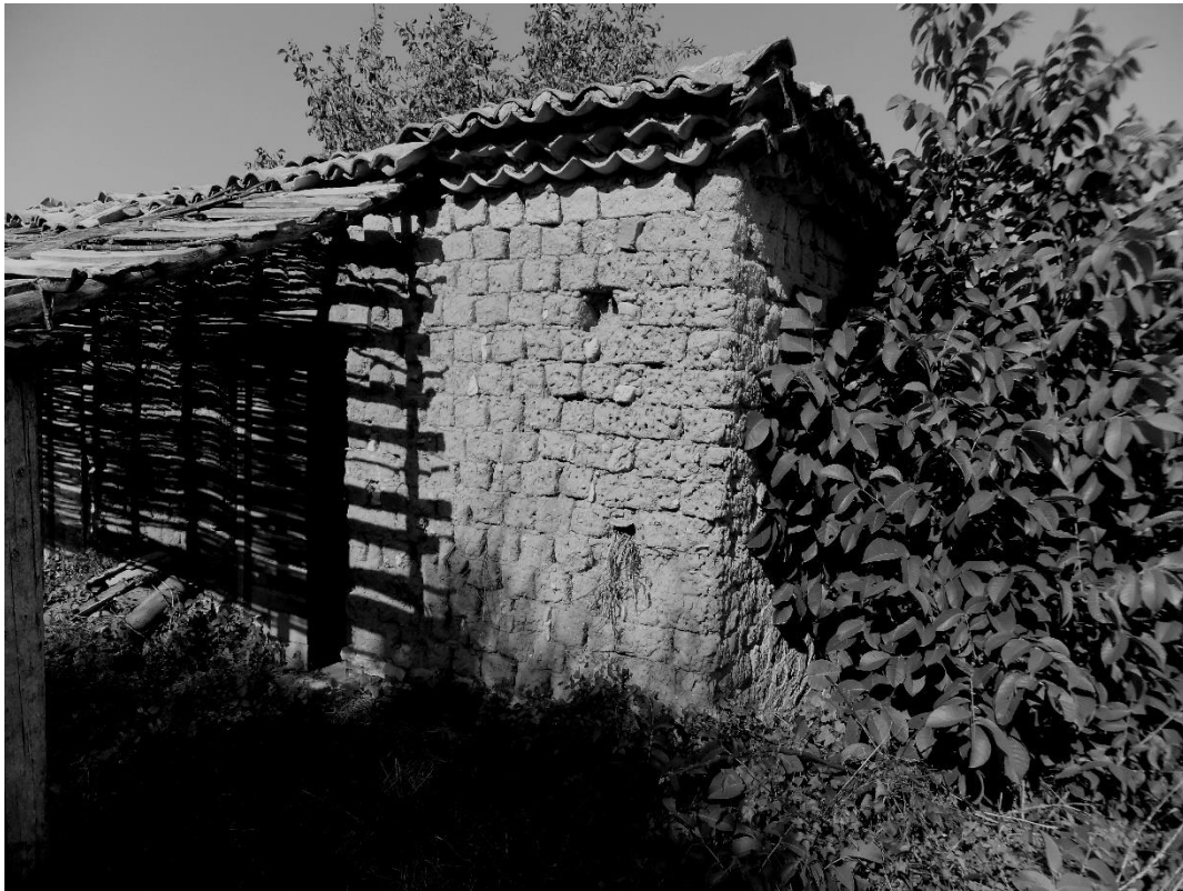
Figure 1. A modern mudbrick structure in Greece that possesses many of the features of the prevailing vernacular methods in the region (photo by author).
