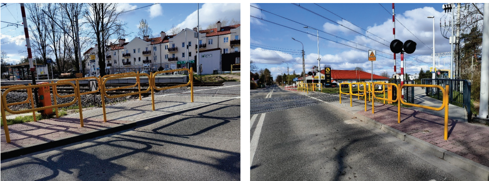
Fig. 7. View of level crossing No. 3 from STOP line.
