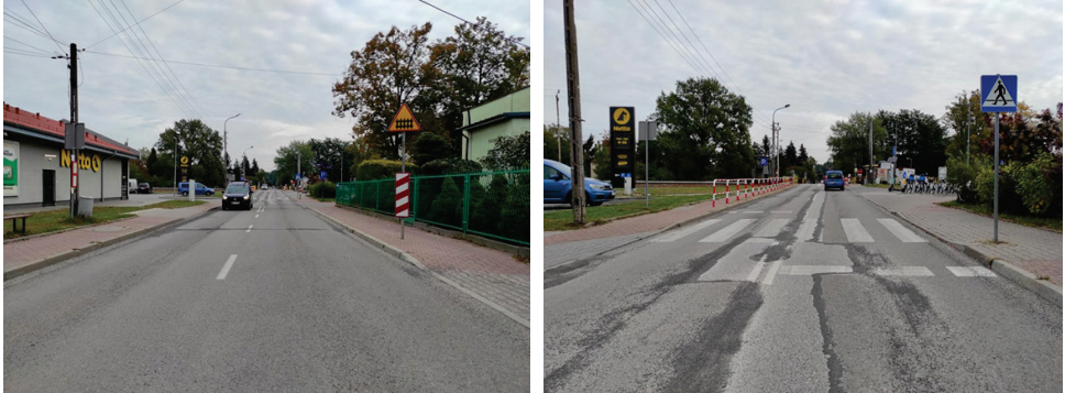
Fig. 5. View of level crossing No. 3 direction A (left 100 m, right 60 m)
